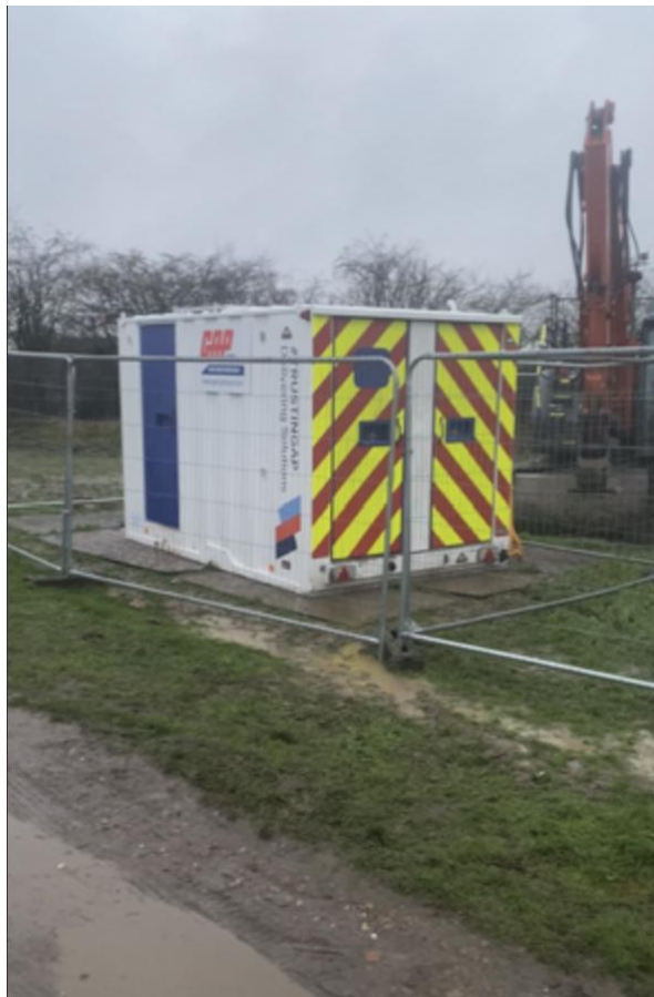
P16 Compound – Place next to Bridleway - Welfare cabin door opening onto public bridleway on metal sheets placed to support structure.
