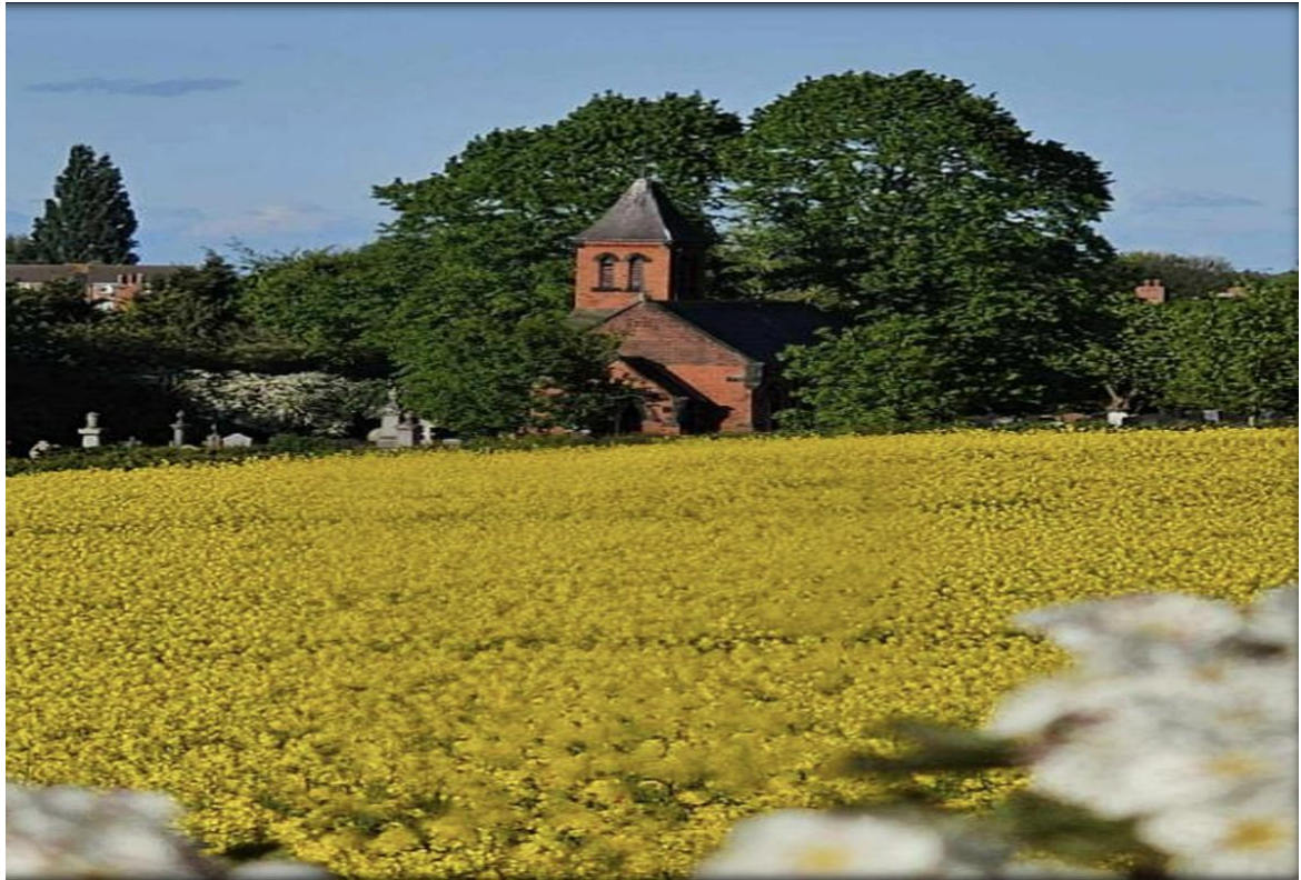
View of Conisbrough Chapel from Park Lane Bridleway proposed entry point.
